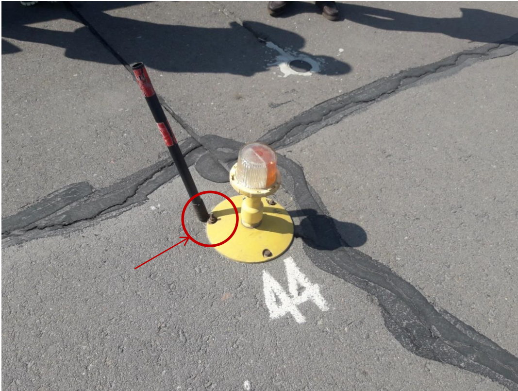
Fig. 7. Photo of the renewed runway edge light No. 44
