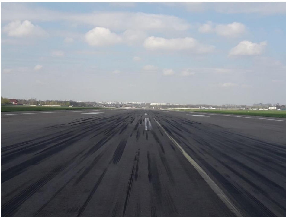
Fig. 8. Photo of the runway centerline marking state
